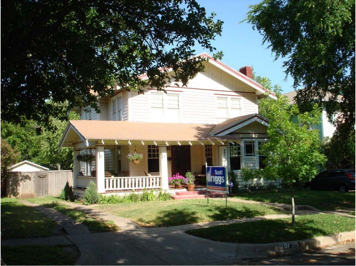
East and partial south elevations.
