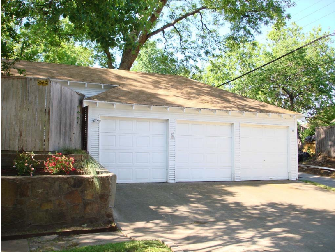
Garage with existing roof.
