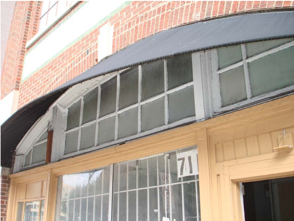
Existing and original transom window. The awning will be removed and not replaced at this time.
