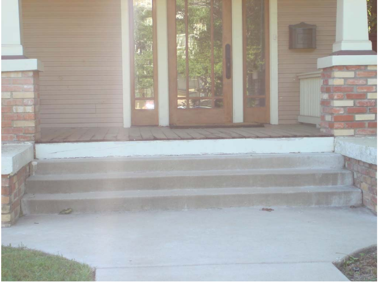
Existing non-historic porch material.
