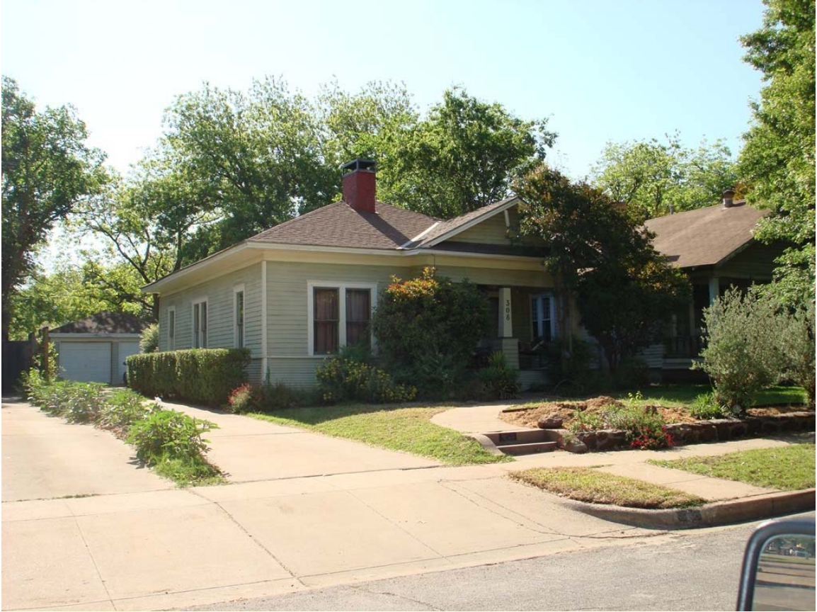
West and partial north façade. Planting area where tree was located is next to the steps/sidewalk.
