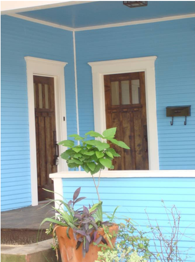
Door and door hardware installed without a Certificate of Appropriateness.
