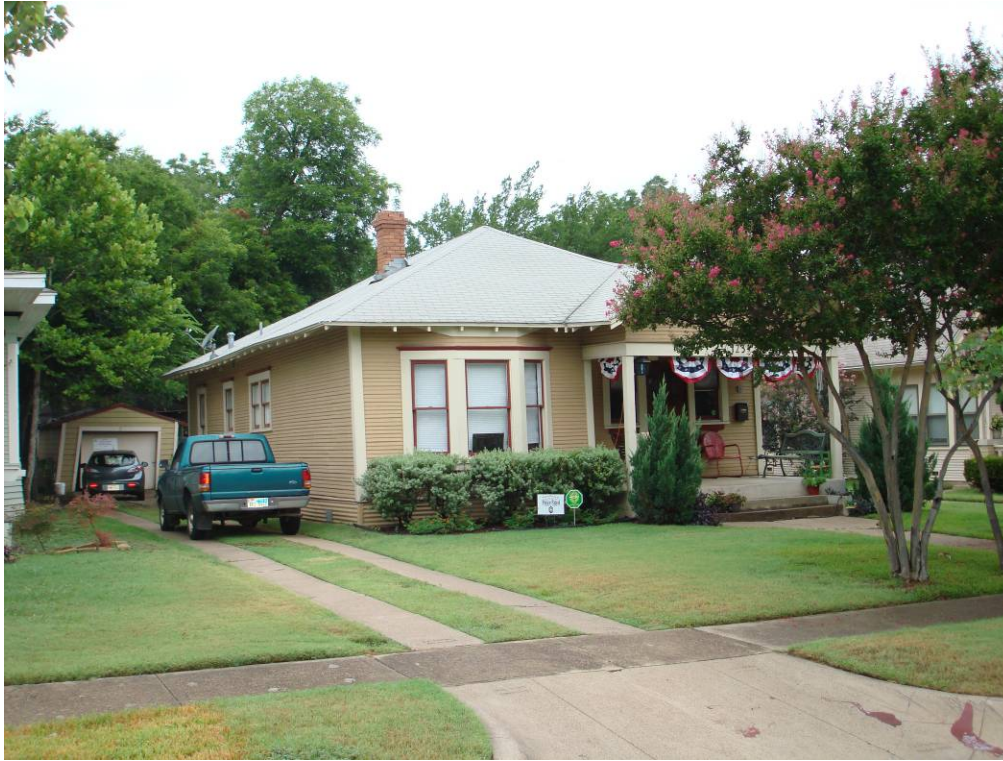
Front (west) elevation of main structure.
