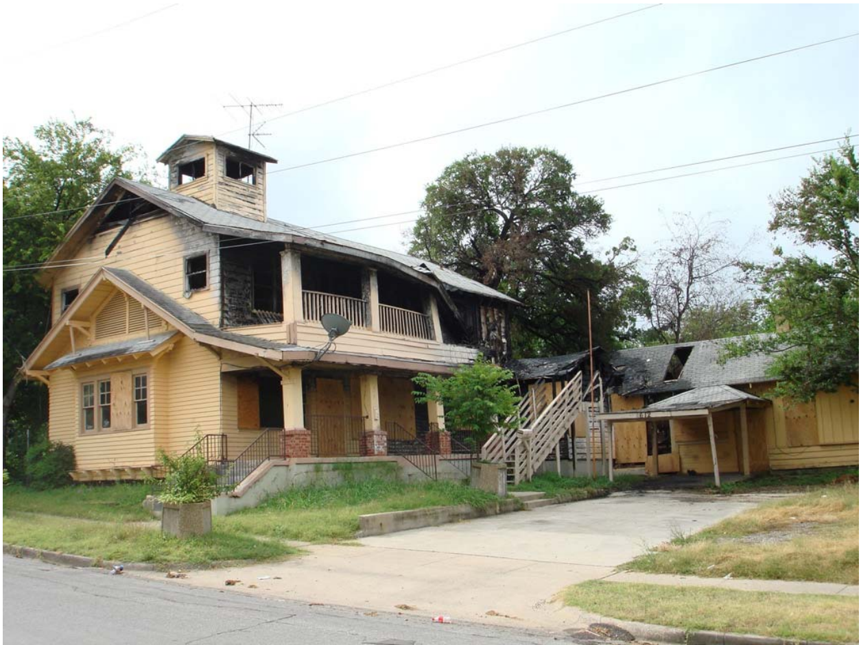
North and partial west elevations.
