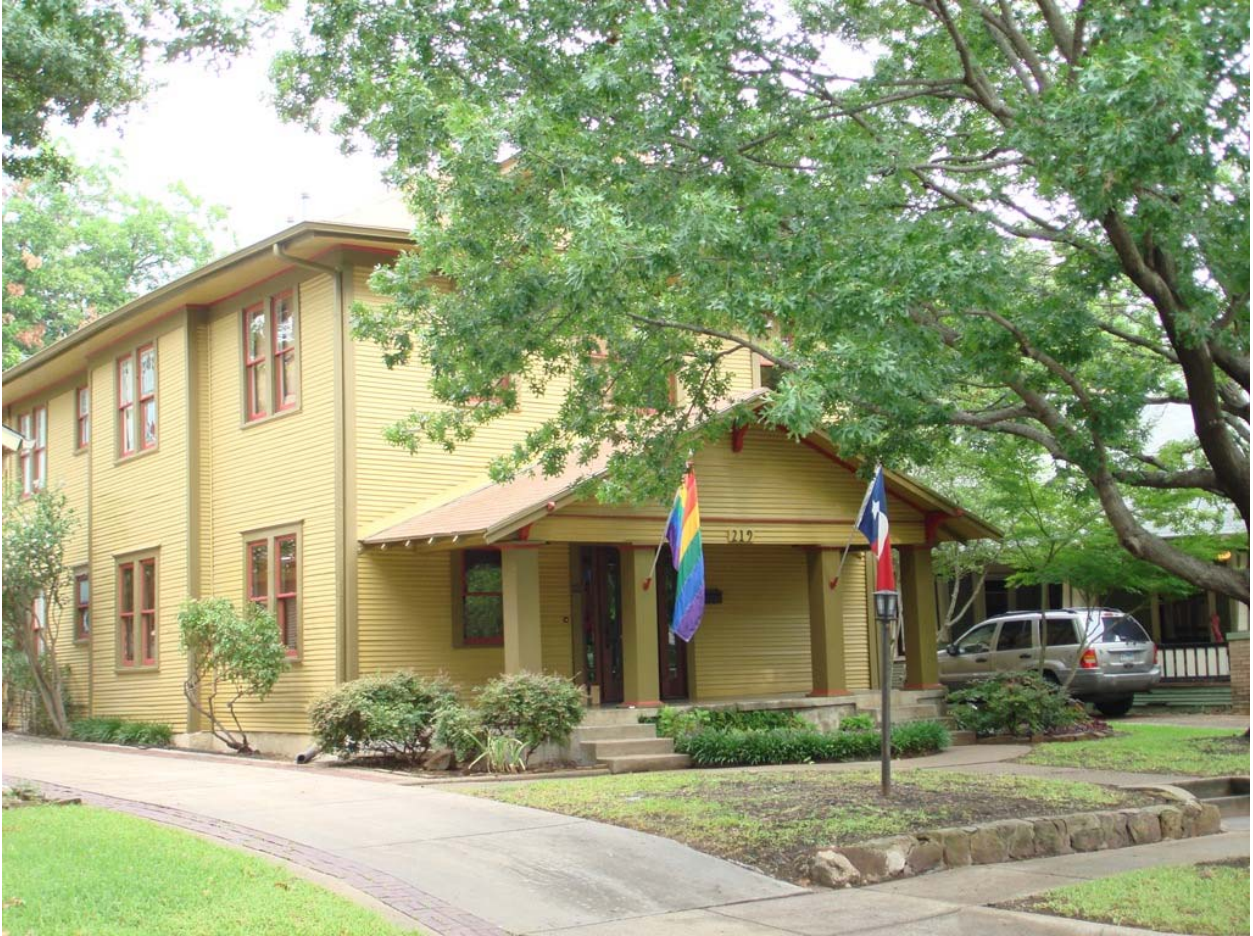
East and partial south elevation.
