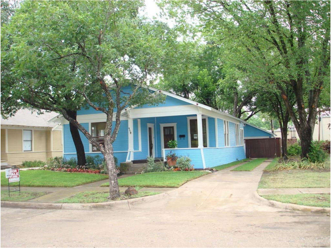
East and partial south elevations.
