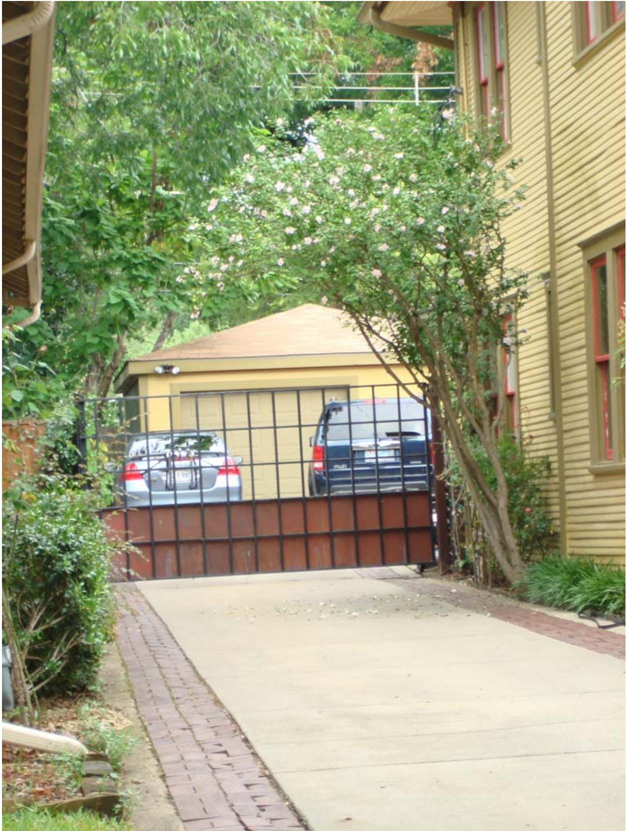
Existing accessory building.
