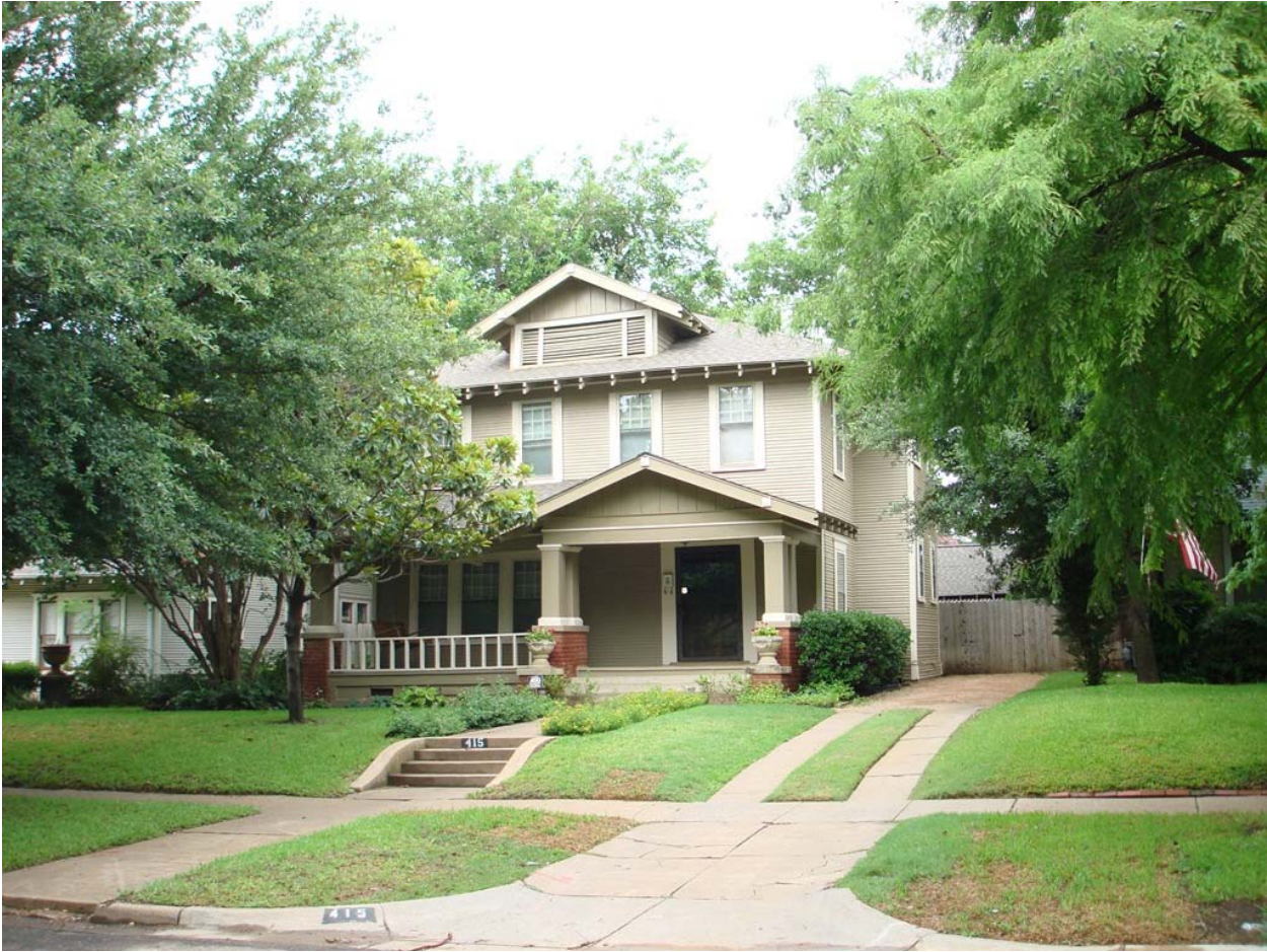
East and partial south elevations.
