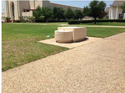
Existing historic drinking fountain in Esplanade, detail
