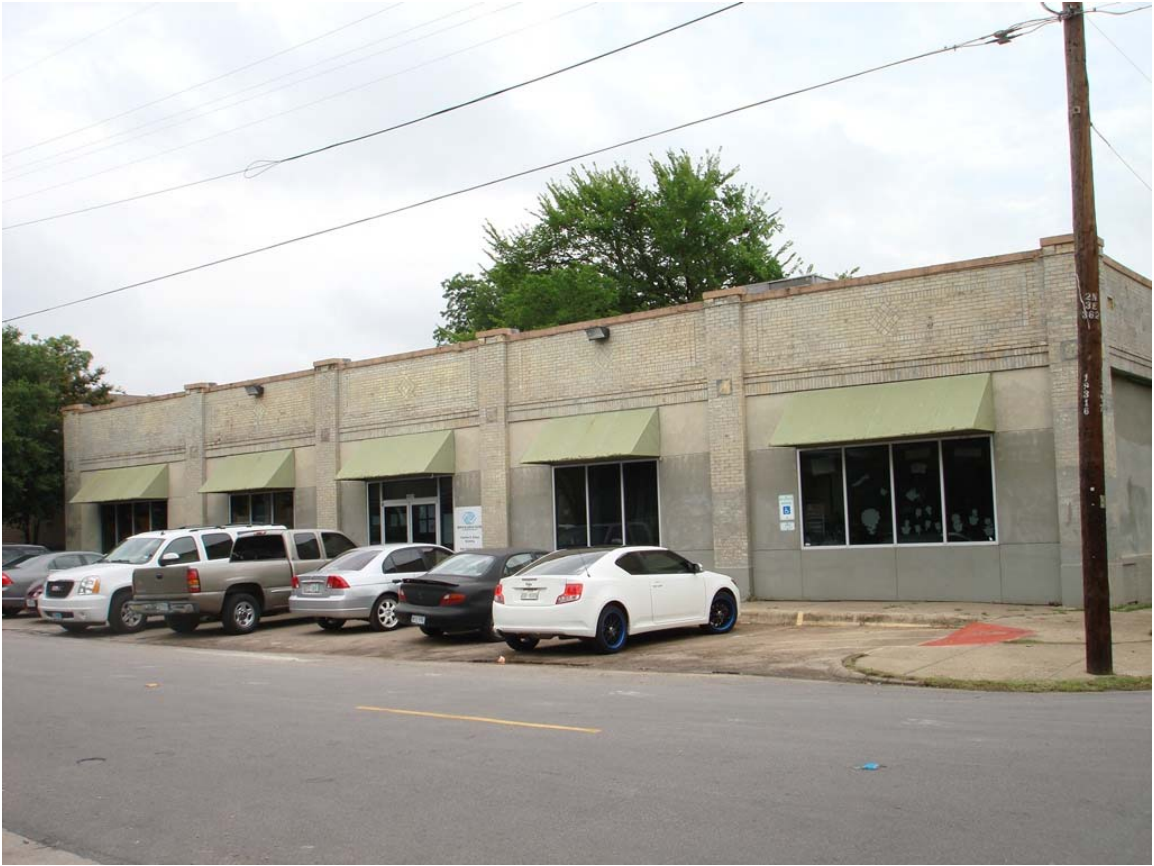
North elevation. Entry to be replaced is located in the middle bay.
