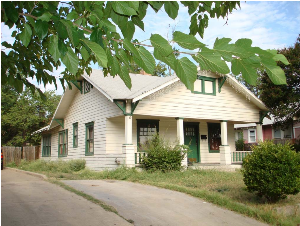
East and partial south elevations.
