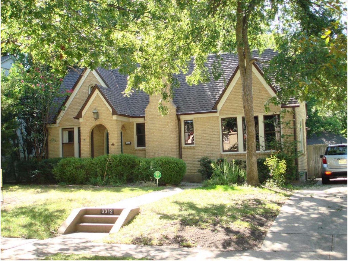
North elevation of main structure.
