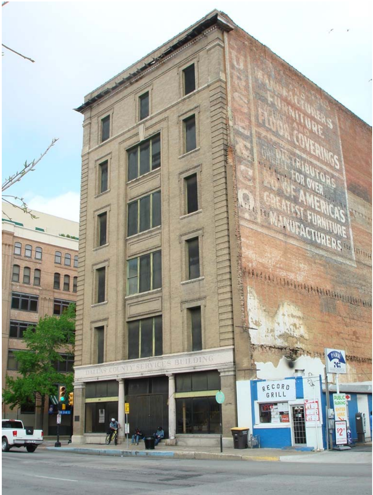
South and partial east façades.
