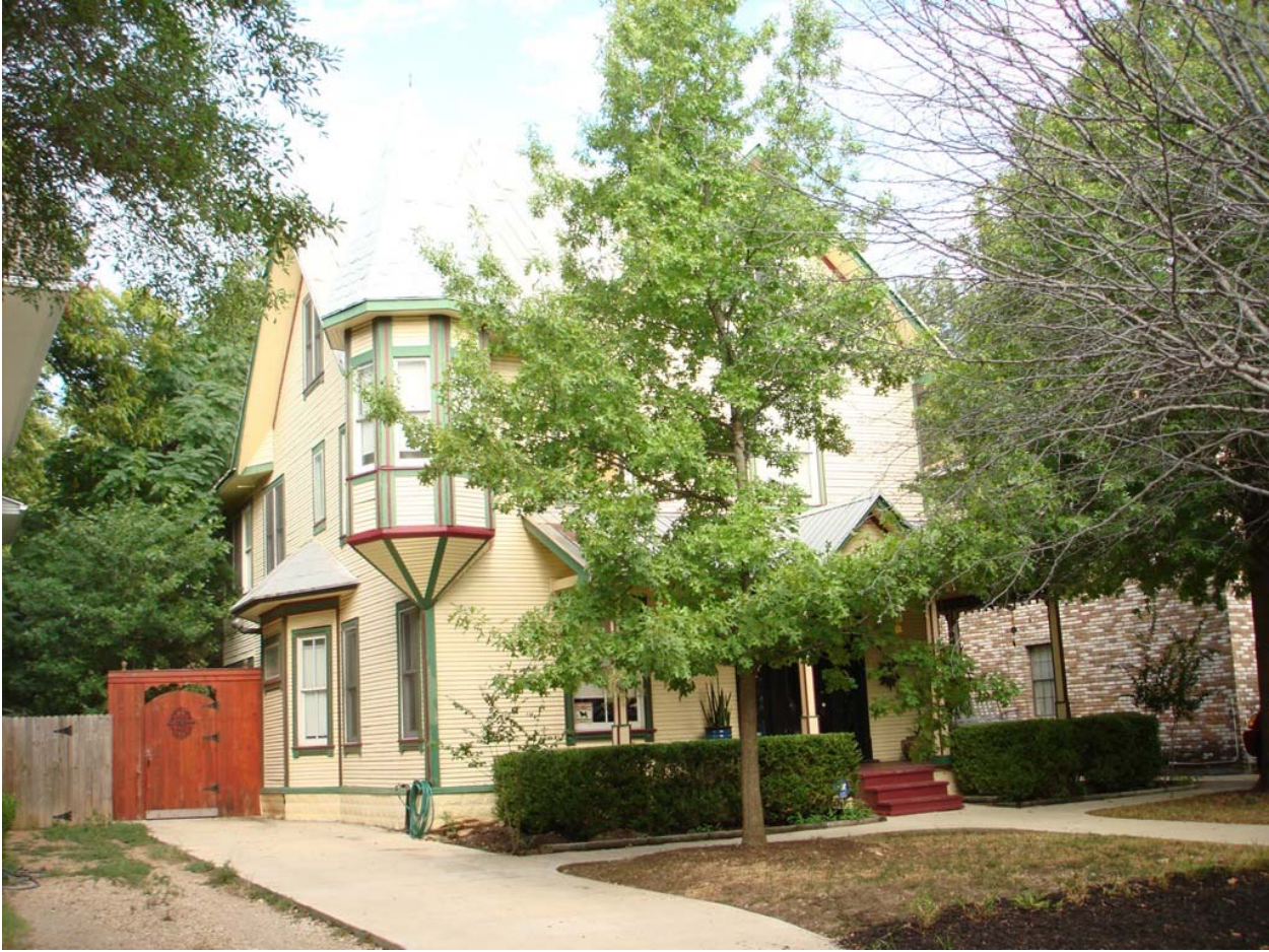
East and partial south elevations.
