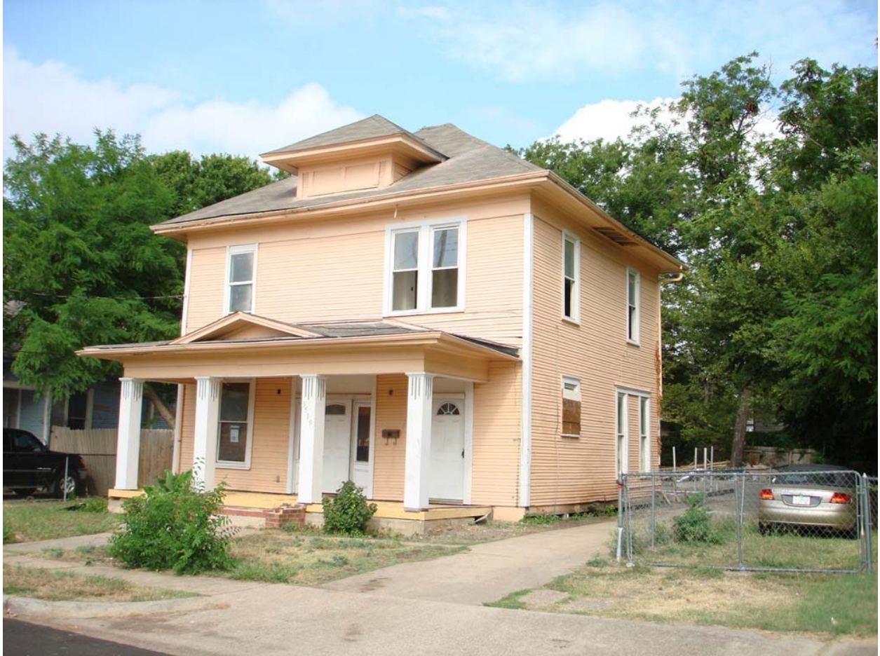
South and partial east elevation.
