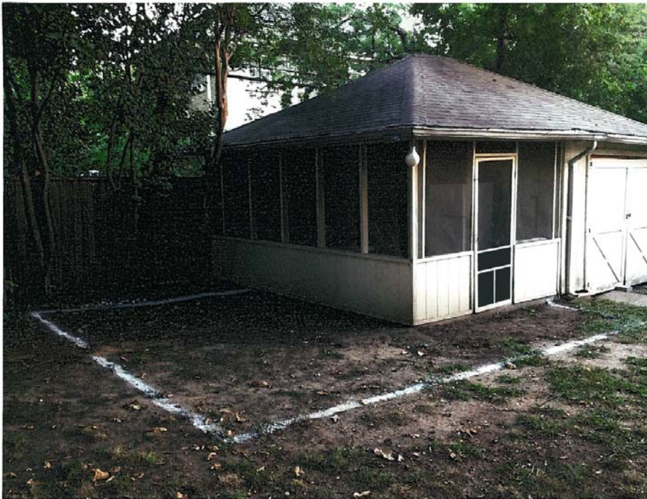
North and east elevation of existing structure. The white stripe indicates the proposed location of the addition.
