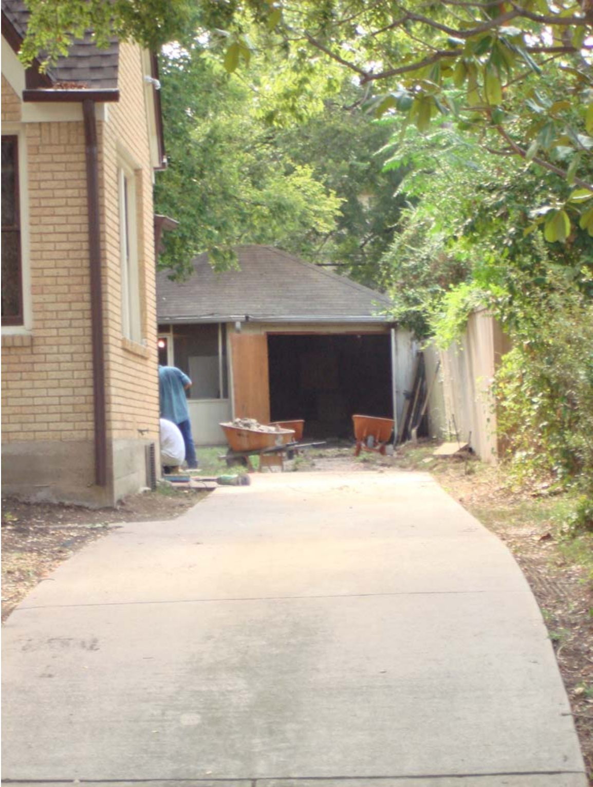
View of existing structure from the street.
