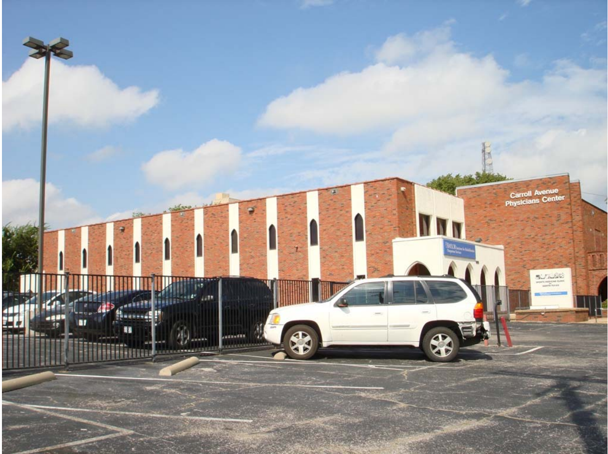
South and partial east elevations.
