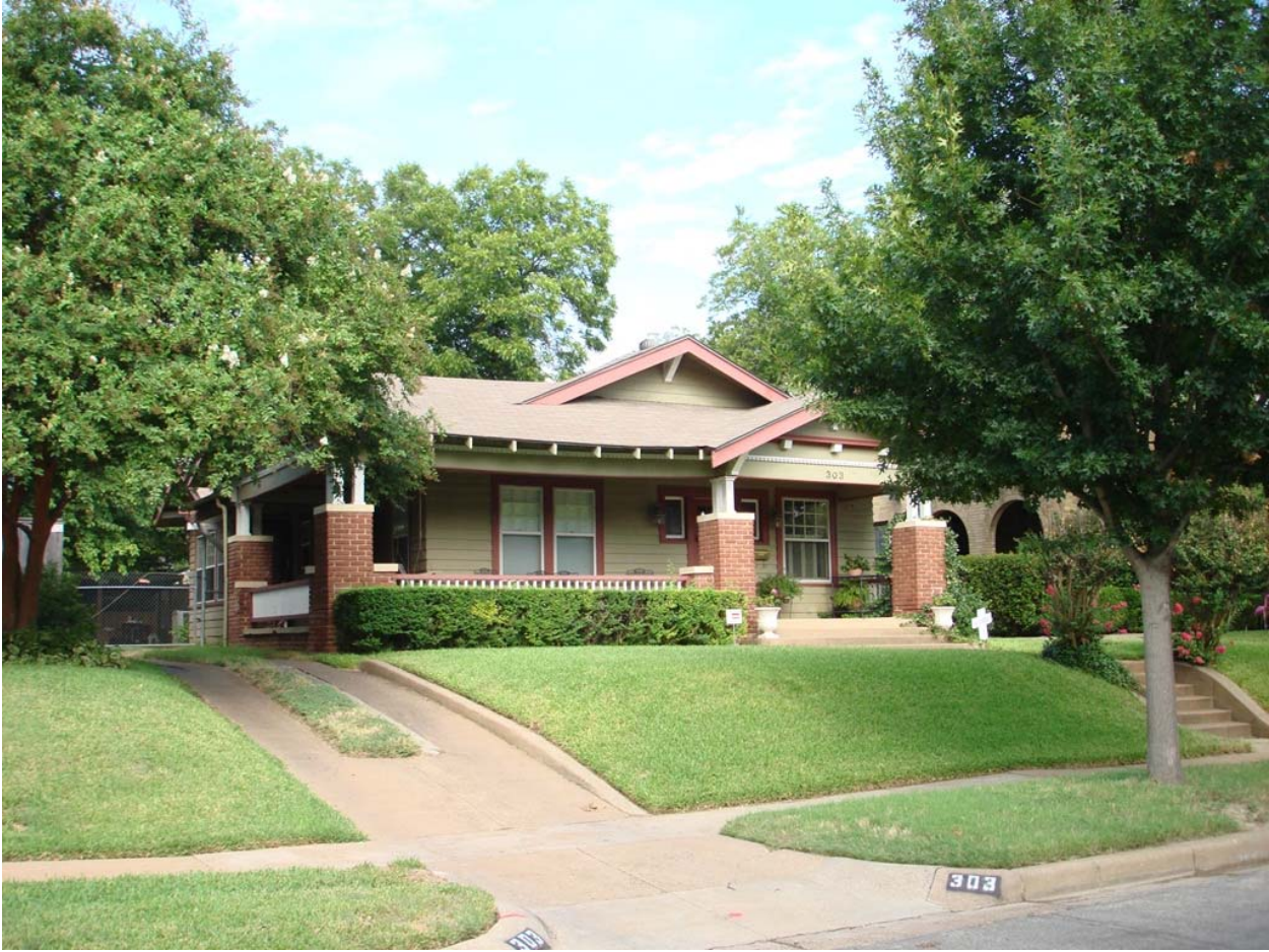
East and partial south facades.
