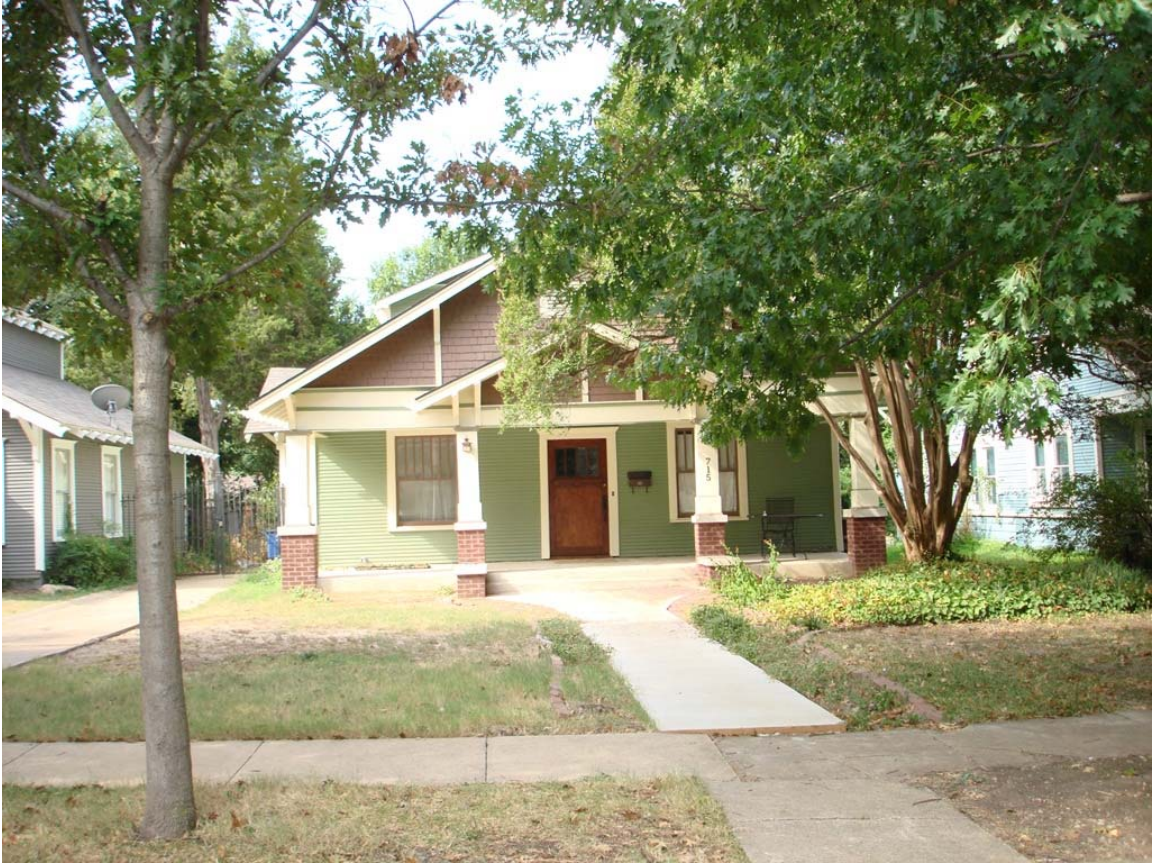
East elevation showing existing landscaping condition.
