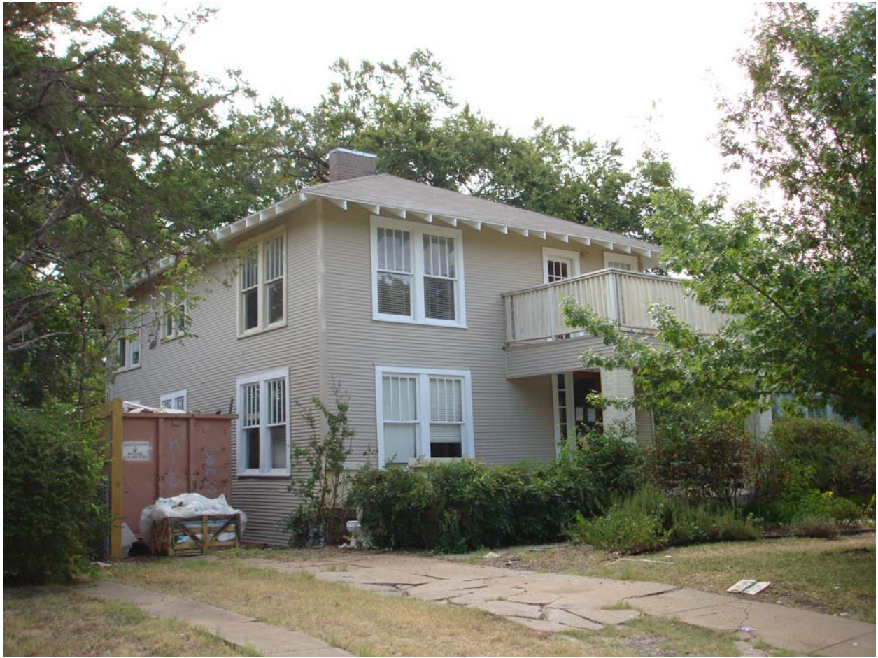
West and partial north elevations.
