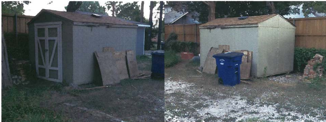
WOOD FRAME SHED, TO BE REMOVED
