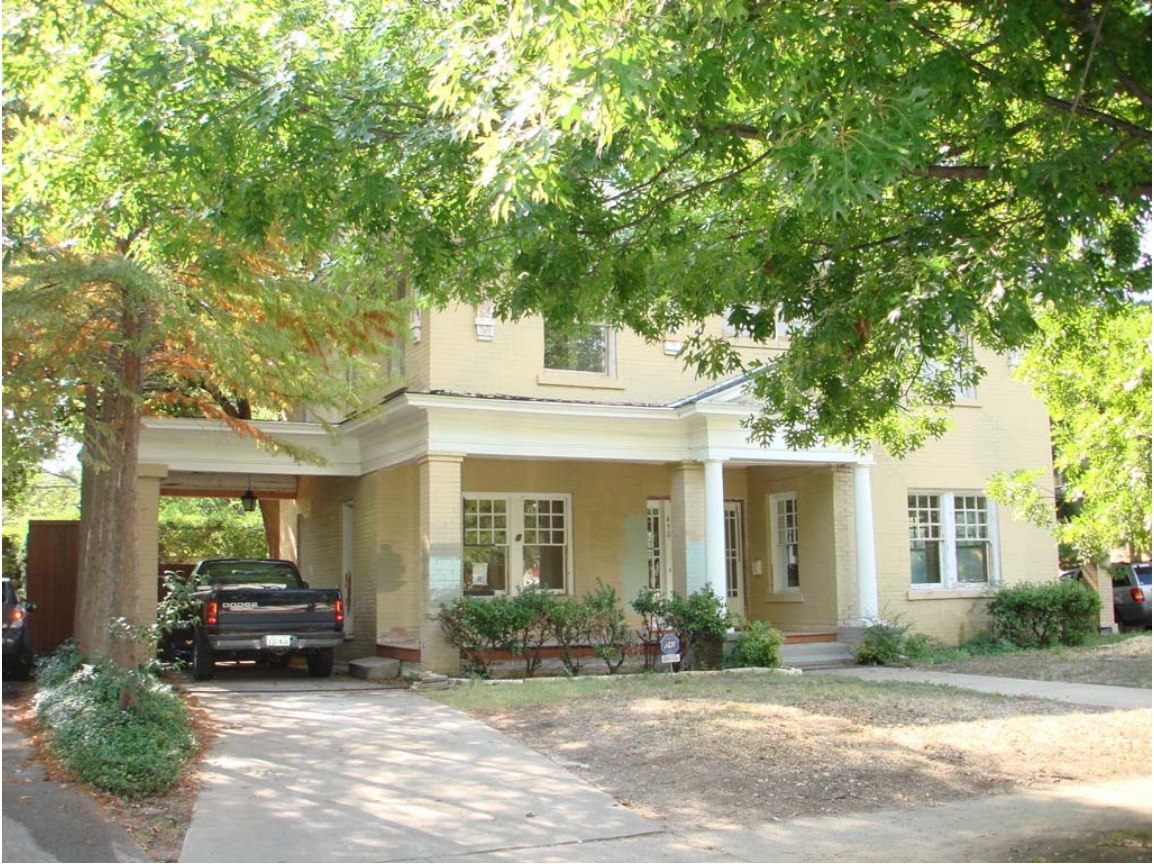
North and partial east elevations.
