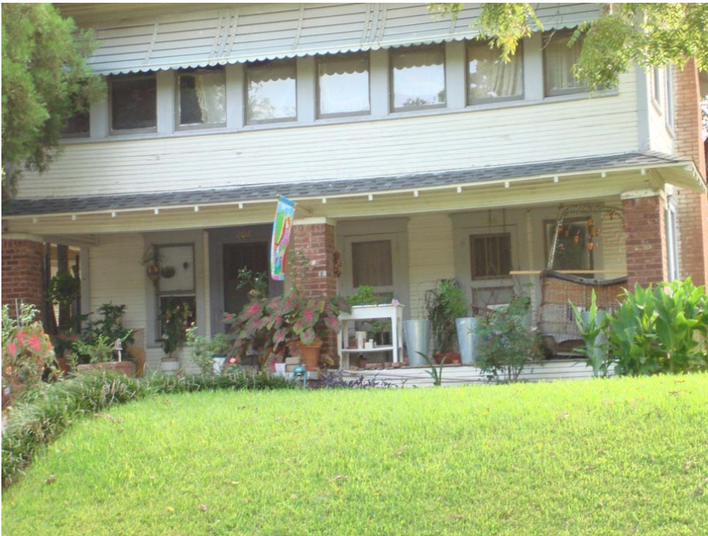
Close up of three existing door openings.
