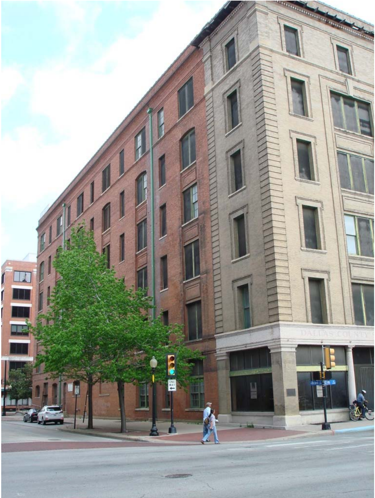
Partial south and west facades.
