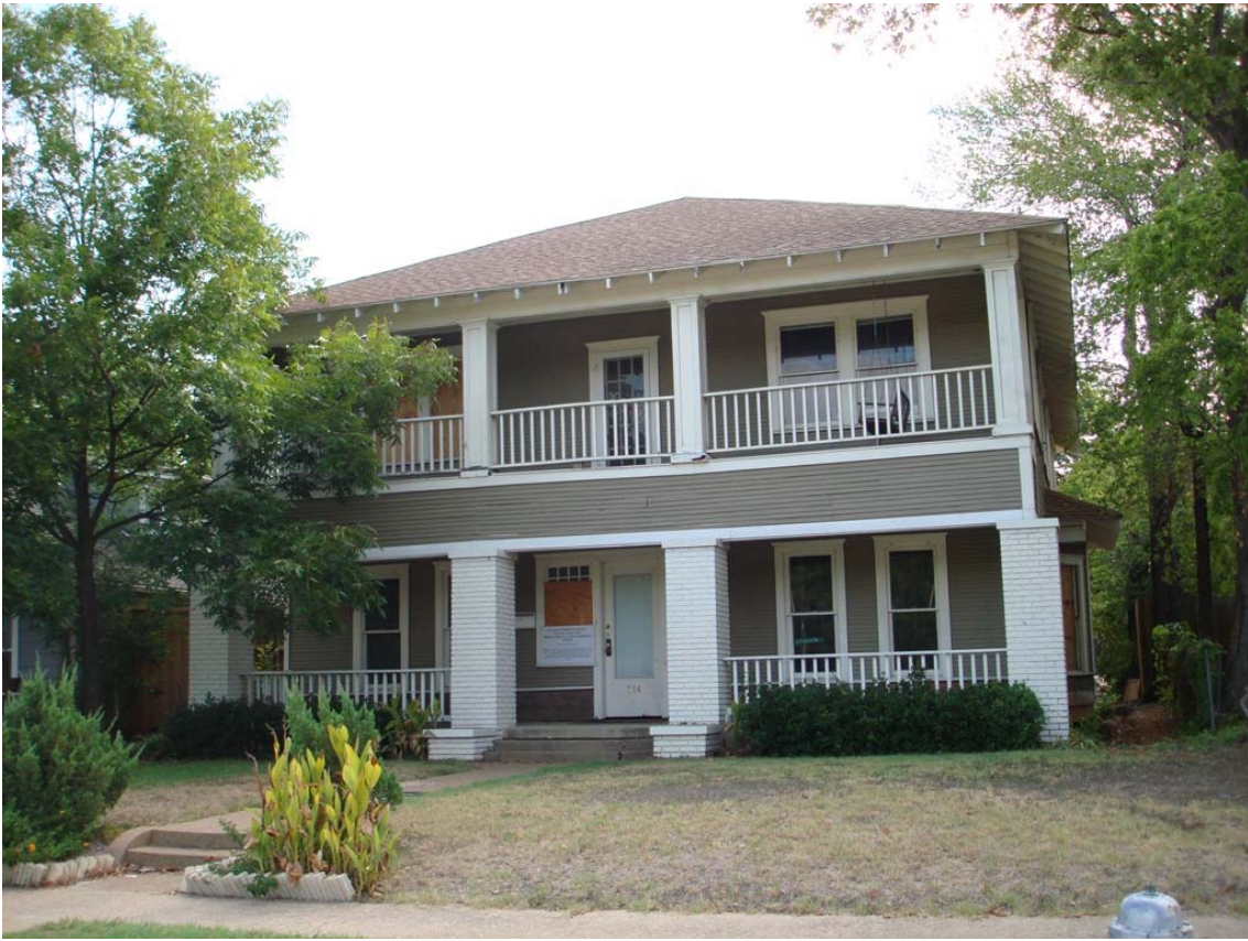
West (front) and south side elevations.
