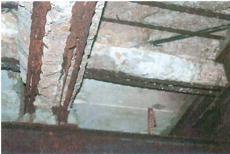
19. SLAB AND BEAM REINFORCING UNDER SIDEWALK.
