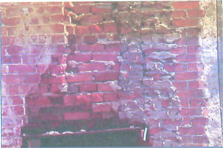
13. S.W. CORNER OF BUILDING
