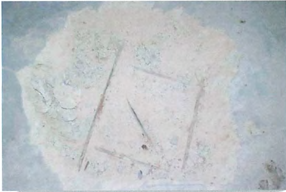
1. SECOND FLOOR SLAB REINFORCING.
