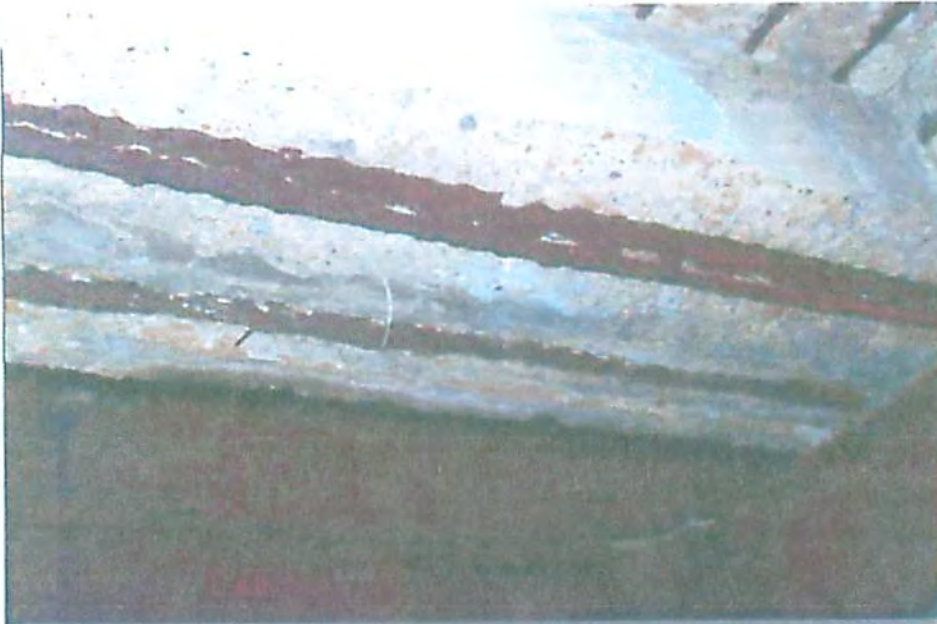
17. BEAM UNDER SIDEWALK.
