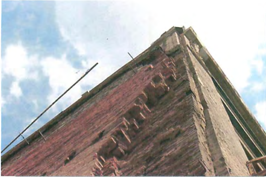
16. WEST SIDE OF BUILDING
