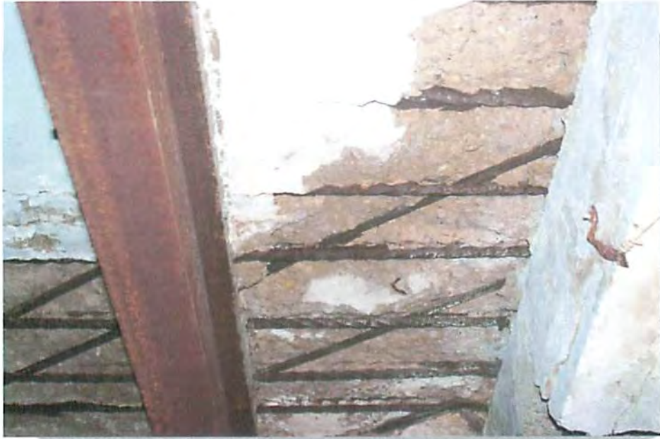
18. SLAB REINFORCING UNDER SIDEWALK.
