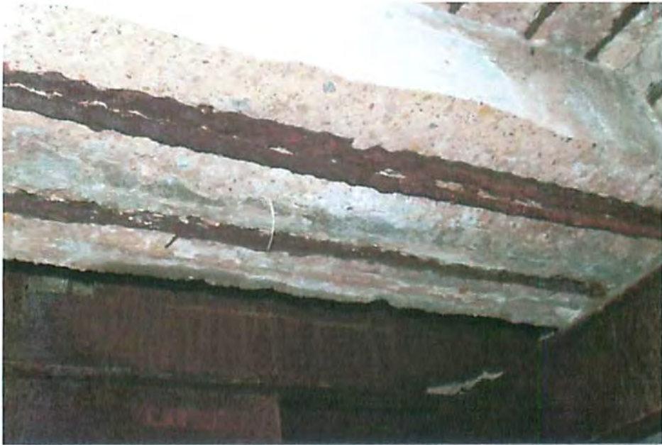
17. BEAM UNDER SIDEWALK.
