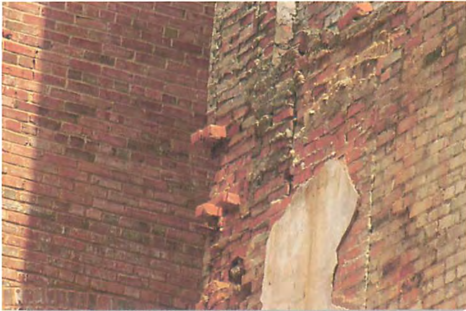
14. S.W. CORNER OF BUILDING
