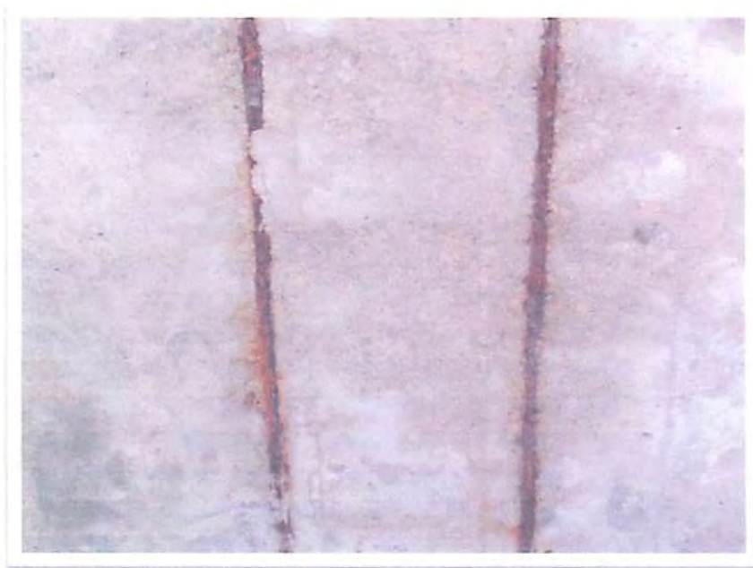
TYPICAL, EXPOSED SLAB REINFORCEMENT. -P7
