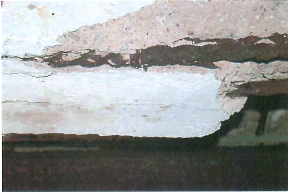
20. BEAM UNDER SIDEWALK.
