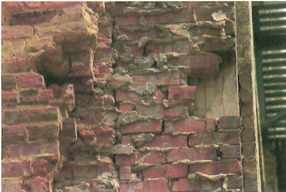
15. S.W. CORNER OF BUILDING
