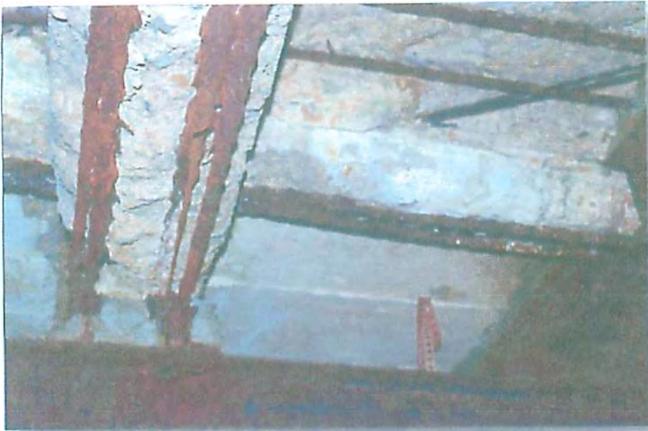
19. SLAB AND BEAM REINFORCING UNDER SIDEWALK.
