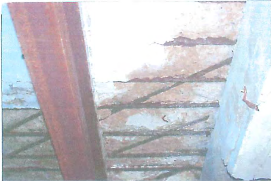
18. SLAB REINFORCING UNDER SIDEWALK.
