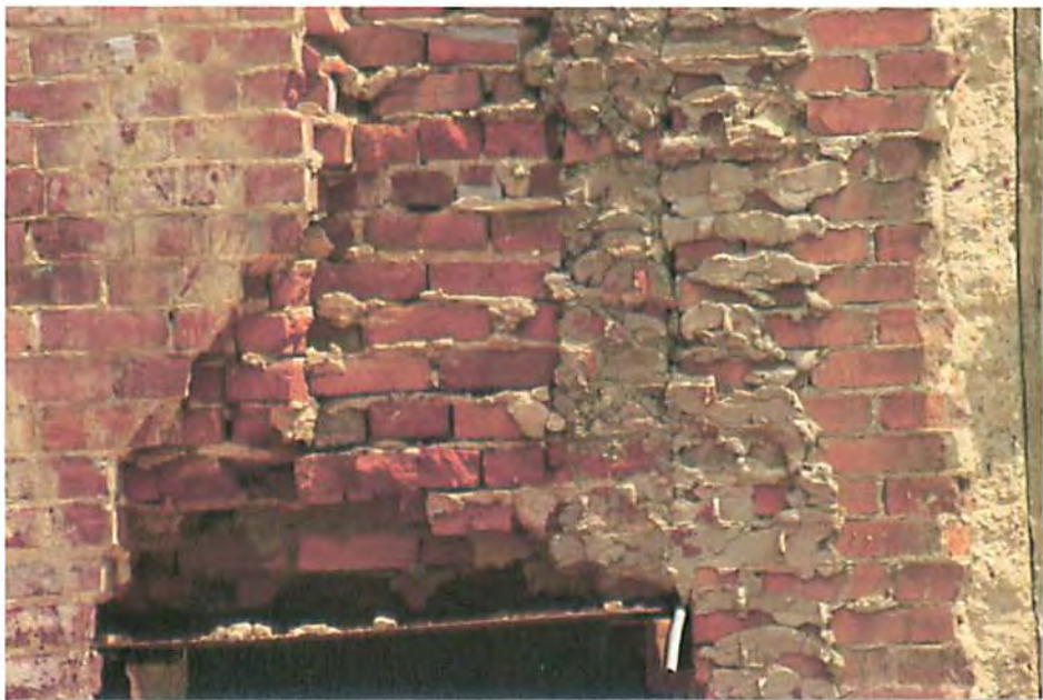
13. S.W. CORNER OF BUILDING
