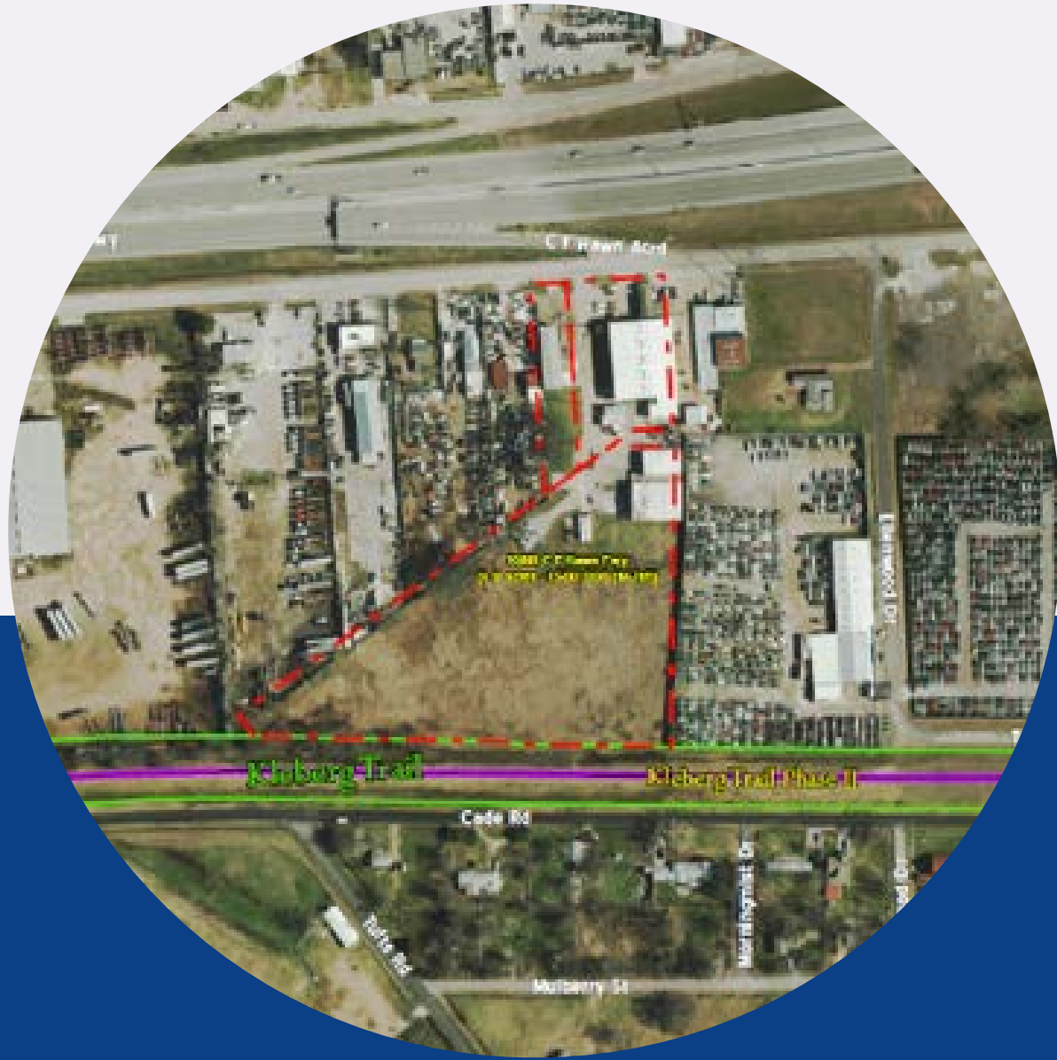
DISTRICT 2 MAINTENANCE SERVICE CENTER
