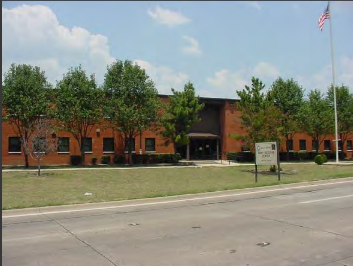
Jules Muchert Army Reserve Center (In progress)
