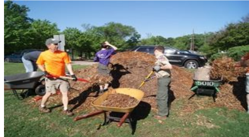
Installation of Mulch at Valley View Park
