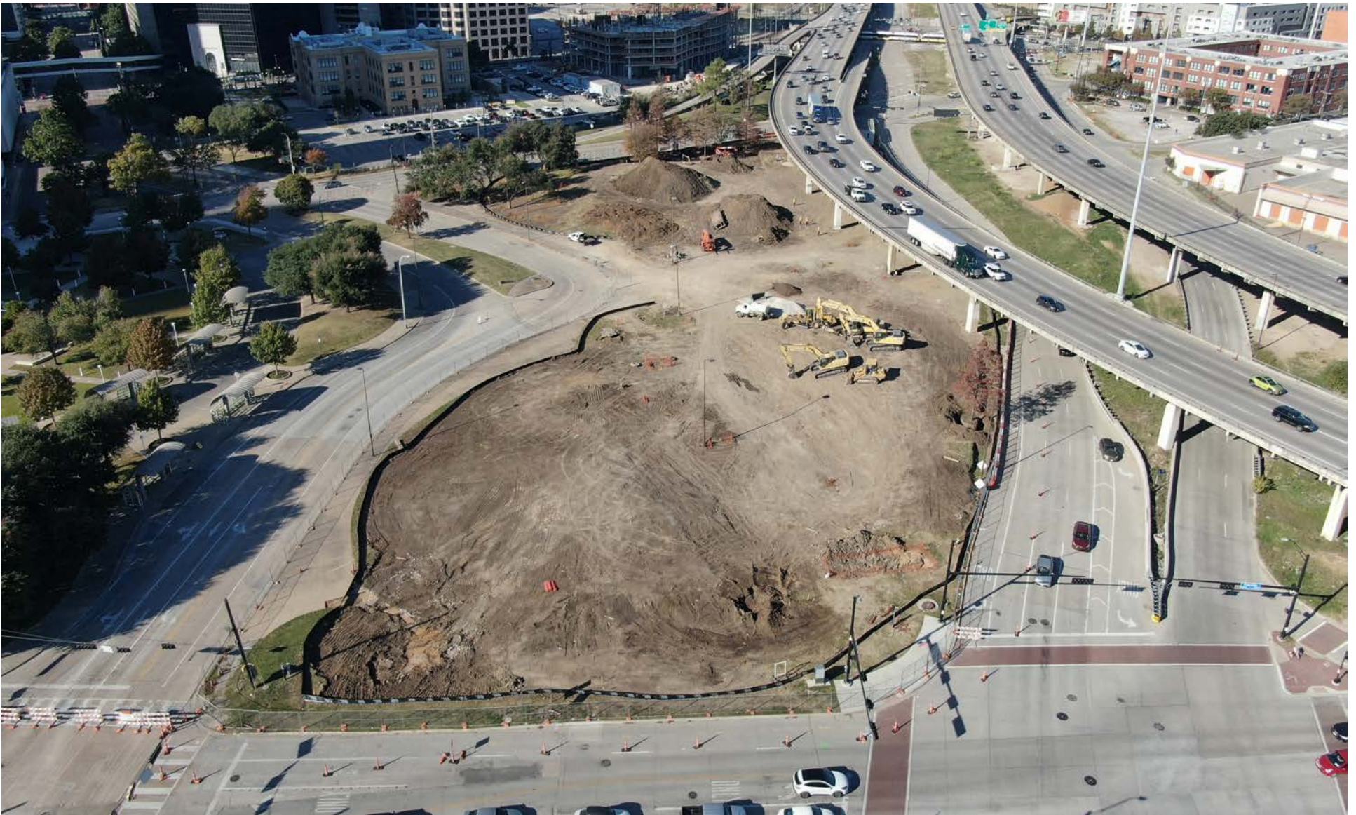
Carpenter Park construction site November 2020
