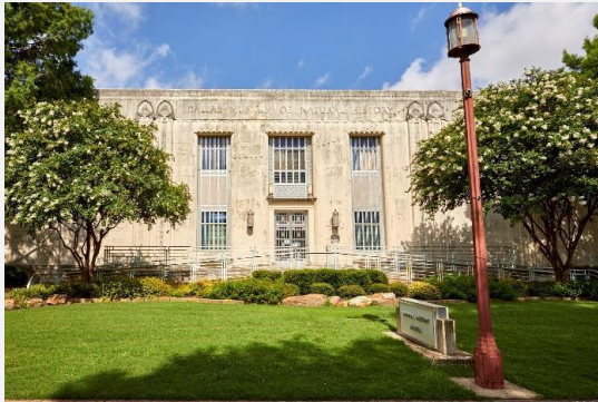
Natural History Building
