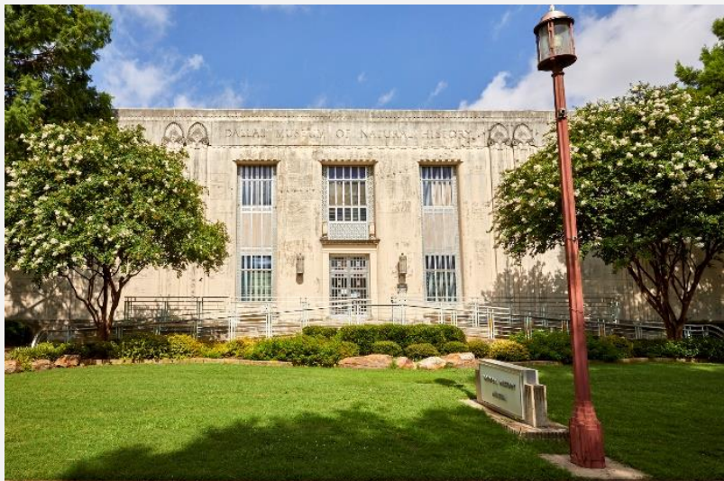
Natural History Building
