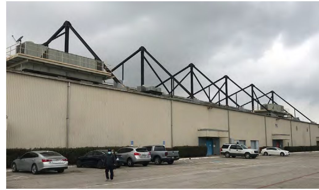
Aircraft Maintenance Hangar (1972-1979)
