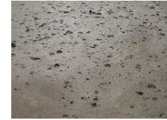
Concrete - Rock Salt Finish
