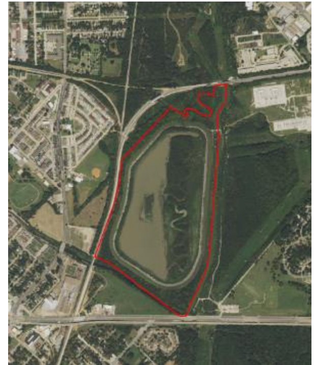
2016: Water level maintained by natural systems
