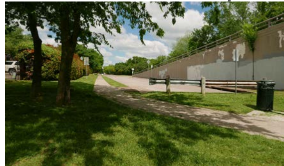
④ Brookside Overpass
