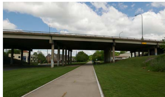
③ Grand Ave Overpass
