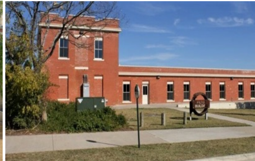
The Filter Building
