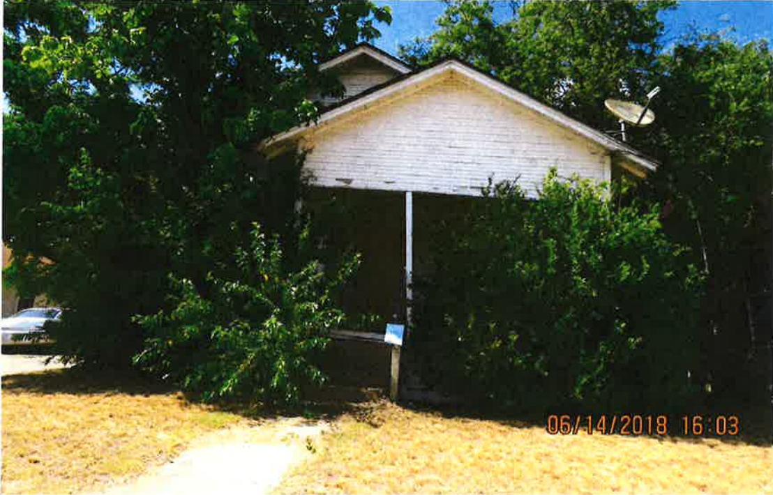
Photo from June 2018 showing front elevation.
