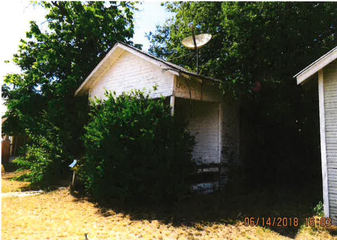
Photo from June 2018 showing front and portion of right side elevation.
