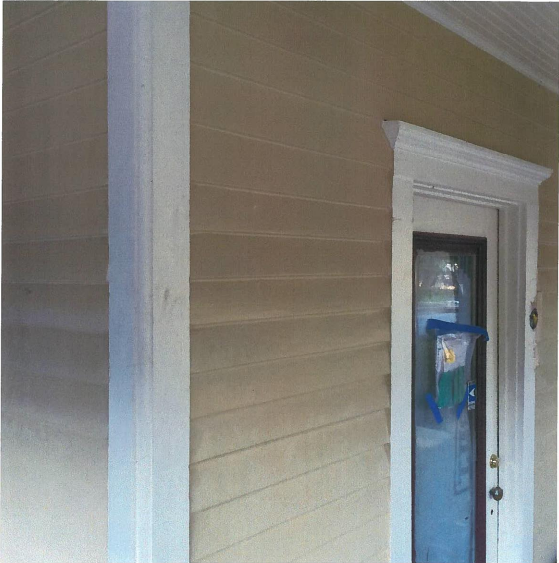
Original siding, front of house
