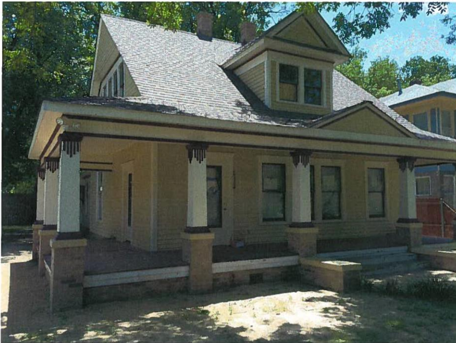
Repainted/restored/ New Roof/restored porch foundation & porch boards etc
