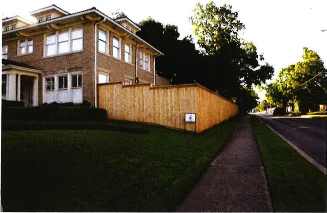
Newly installed fence
