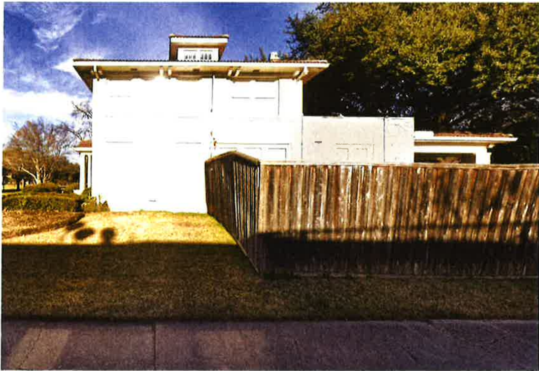
Original fence location
