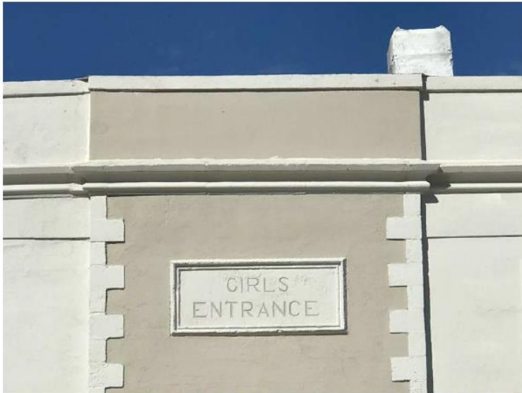
Detail of inset concrete 'GIRLS ENTRANCE' sign at south facade. January 28, 2019.
