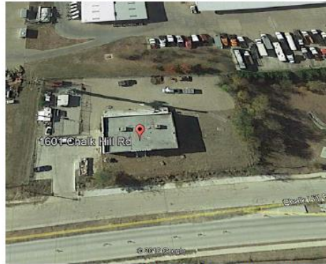
Current aerial view of Eagle Ford School site, showing road construction at Chalk Hill Road currently underway. Courtesy of Google Earth accessed January 28, 2019
