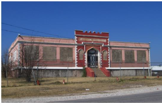
Photograph of Eagle Ford School prior to recent rehabilitation, August 14, 2014.
