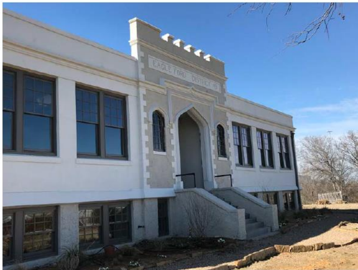
East façade at Chalk Hill Road, looking west. January 28, 2019.
