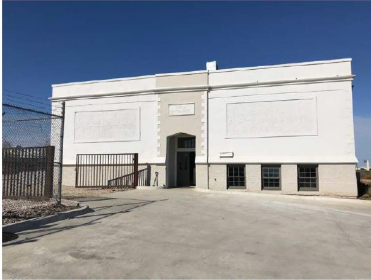
South façade with 'GIRLS ENTRANCE' sign. January 28, 2019
