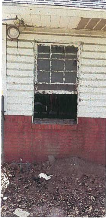
Request #4 – Close up of wood window on rear elevation.
