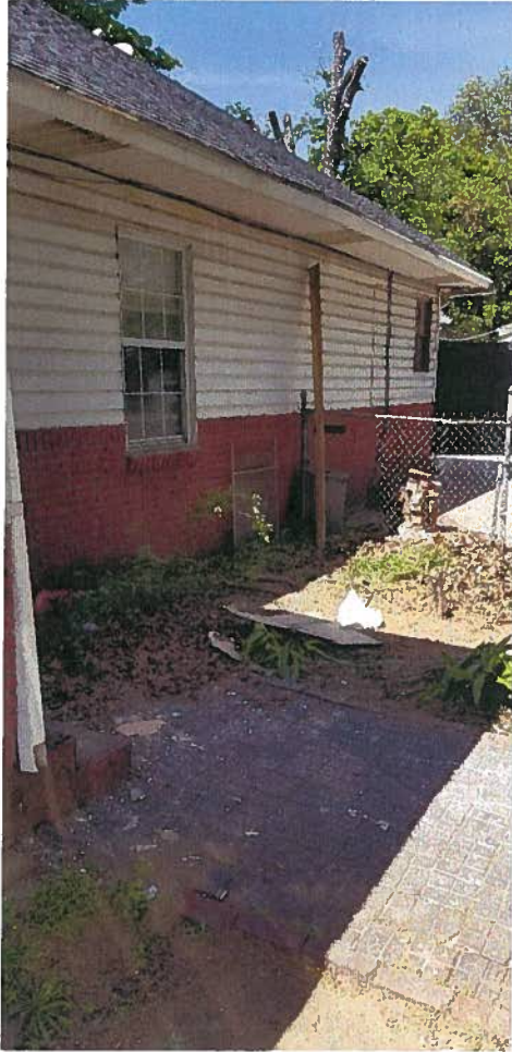
Request #4 – Photo of current vinyl windows on side elevation.
