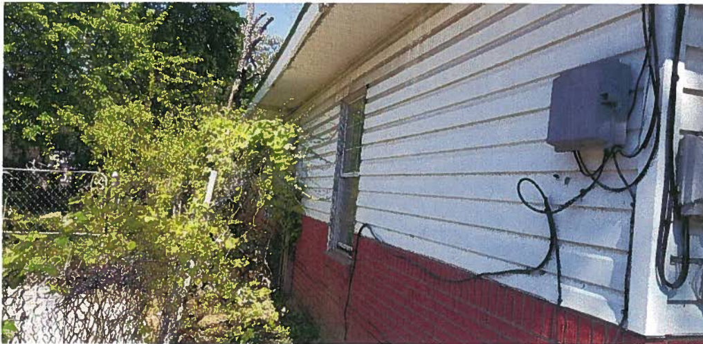
Request #4 – Photo of current vinyl windows on side elevation.
