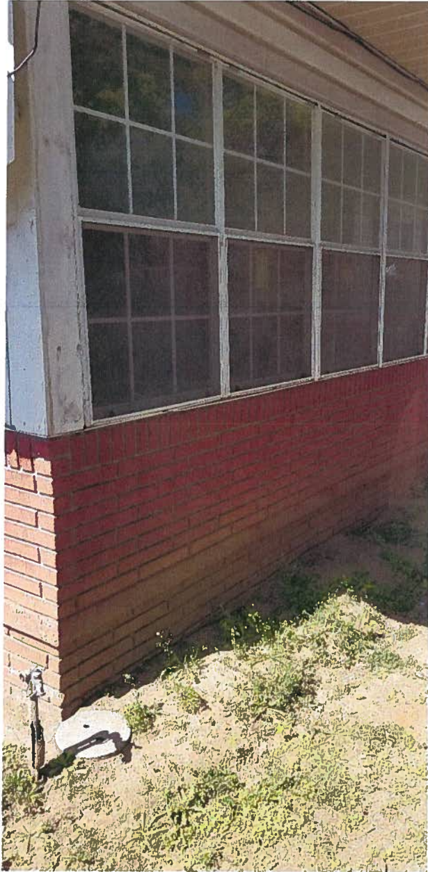
Request #4 – Photo of vinyl windows on side elevation.
