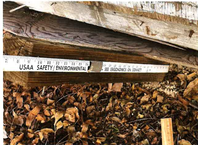
South elevation base @ column location seen at porch decking (no columns existing)
