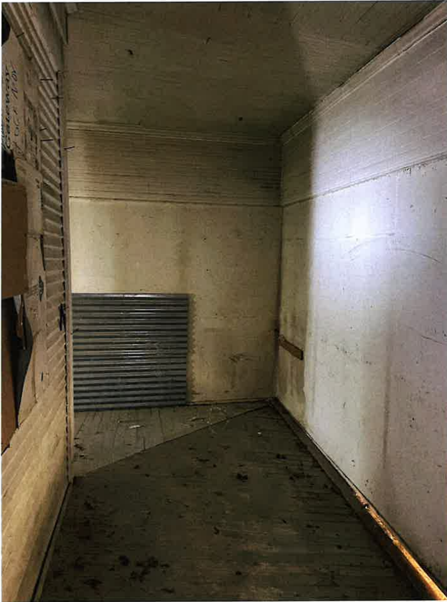
Figure 17 – Partial view of the enclosed wrap-around porch (photograph taken July 25, 2022)
