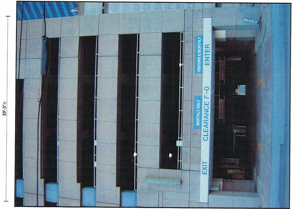
39'-3"± 1'-10"± 1'-10"± 8'-0"± EXISTING SIGNAGE REMOVE EXISTING SIGNS & DISCARD AS REQ'D - VERIFY CONSTRUCTION NOT TO SCALE
