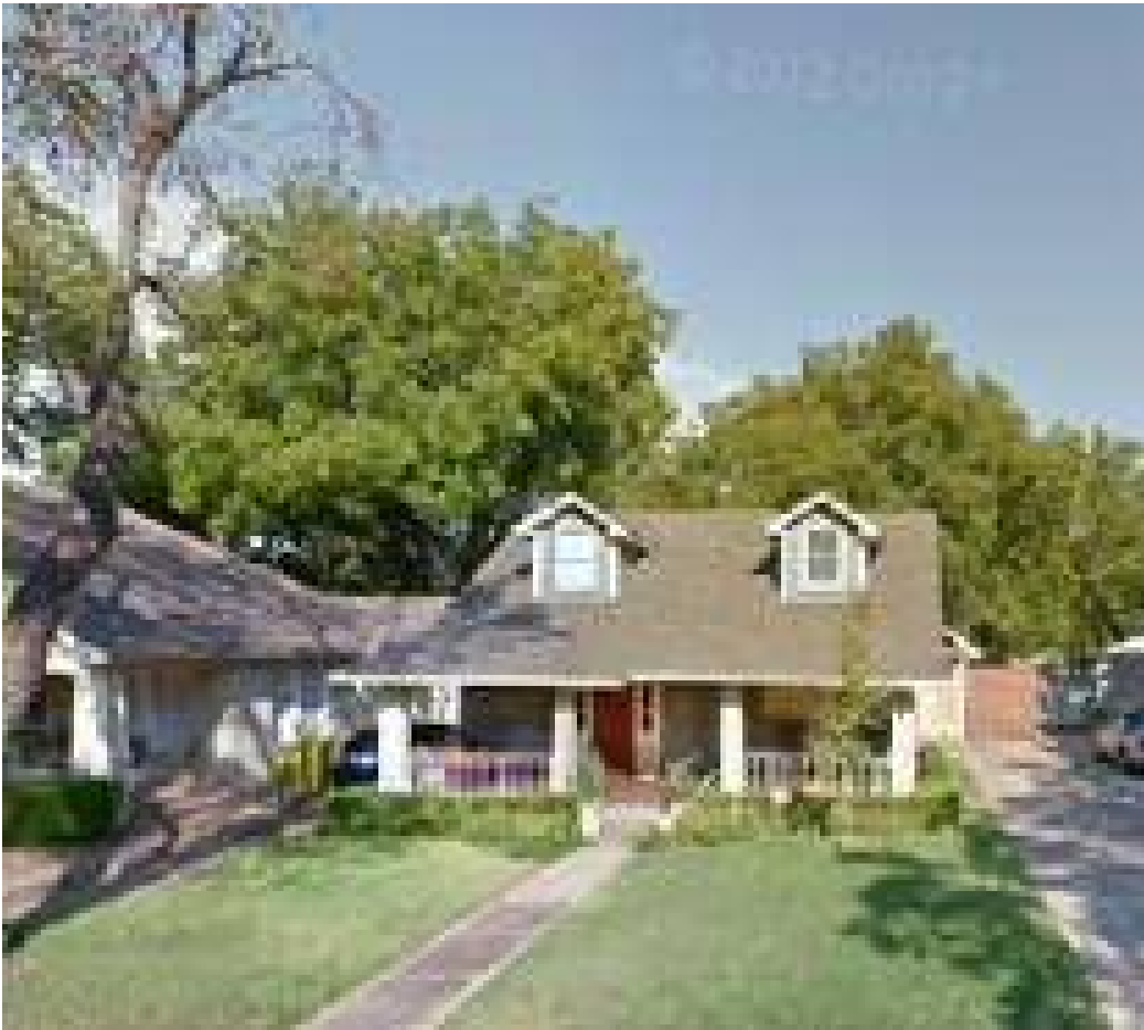
Front façade with original walkway.
