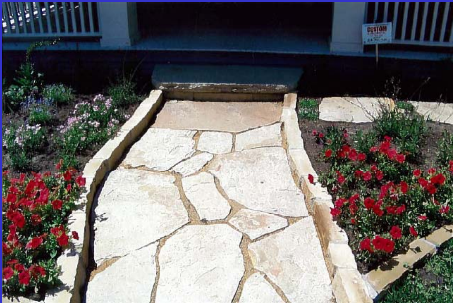
New flagstone installed
