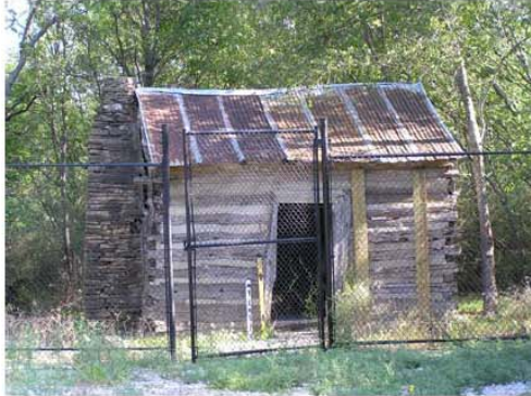
Log cabin with reinforcement, August 2007.
