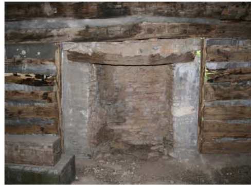
Stone fireplace inside log cabin, February 2008.
