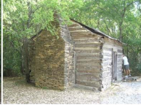
Log cabin, west elevation.
