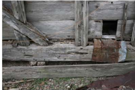
Log barn foundation at crib, February 2008.
