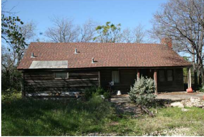
Farmhouse, east façade (facing log cabin), 200.9
