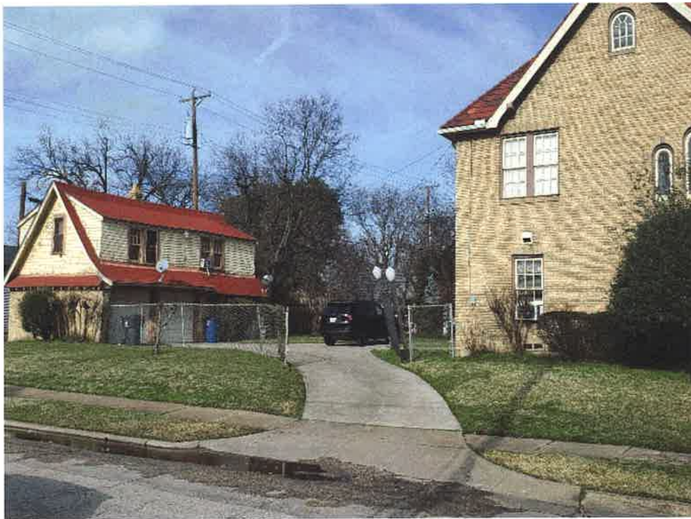
B1: Historic unit at 2601 South Blvd. with an accessory unit in the rear.
