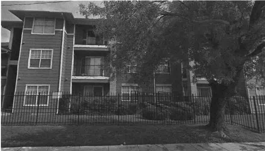
C2: Multi-Family residential units at 2900 Al Lipscomb Way (approximately 250 yards north of 2634 Al Lipscomb Way)—an occupancy of approximately 450 persons
