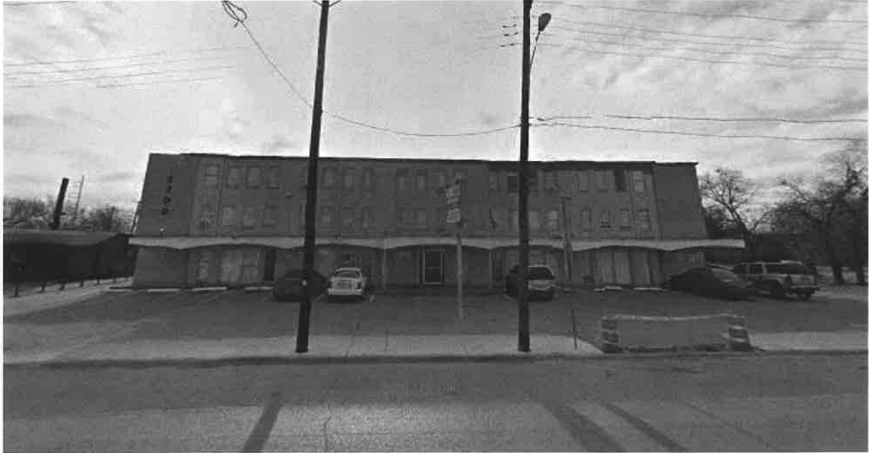
C1: Multi-Family residential units at 2700 Al Lipscomb Way (adjacent to 3624 Al Lipscomb Way)—an occupancy of approximately 100 persons
