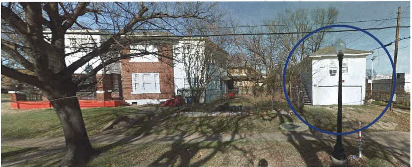
B5: Historic unit at 2402 South Blvd. with an accessory unit in the rear (listed as a Mother-in-Law Apartment).
