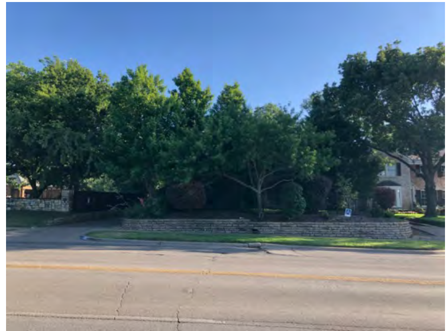
6725 Gaston- 3' Retaining Wall and 4' Iron Fence
