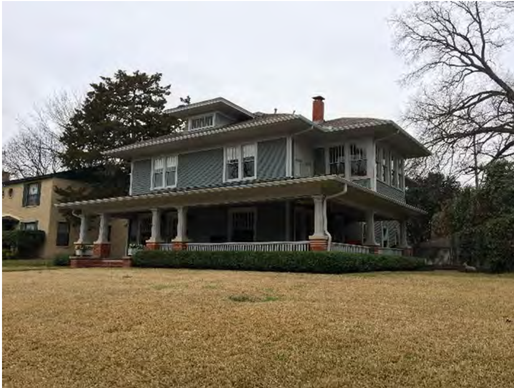
Existing main structure from front yard
