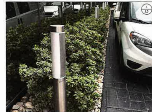
EXISTING 4'-6" WIDE PLANTING AREA AT BUILDING FOUNDATION
