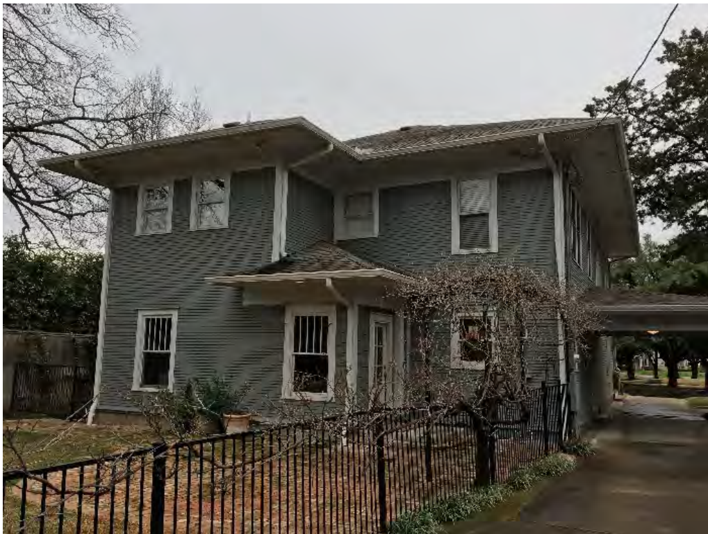
Existing main structure from rear yard.
