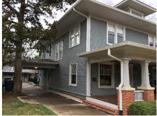
View of existing historic front porch.
