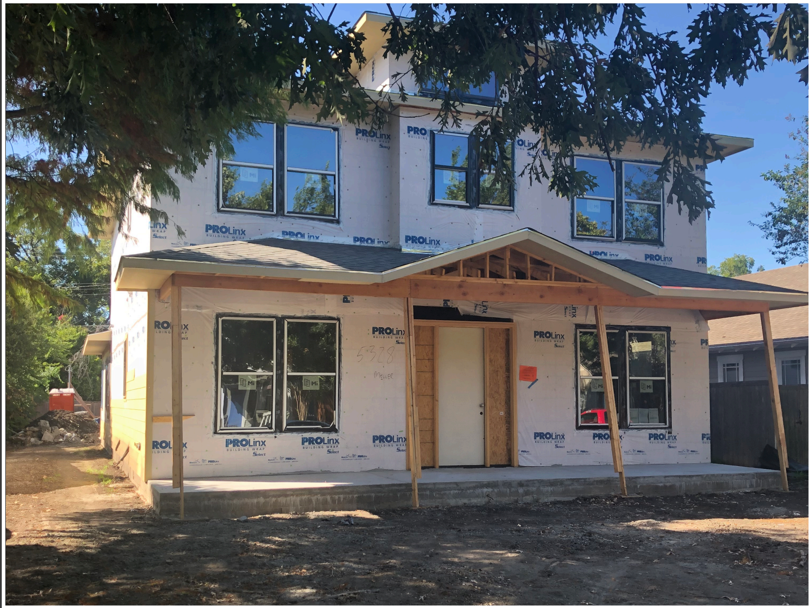
CURRENT EXISTING SITE CONDITION
