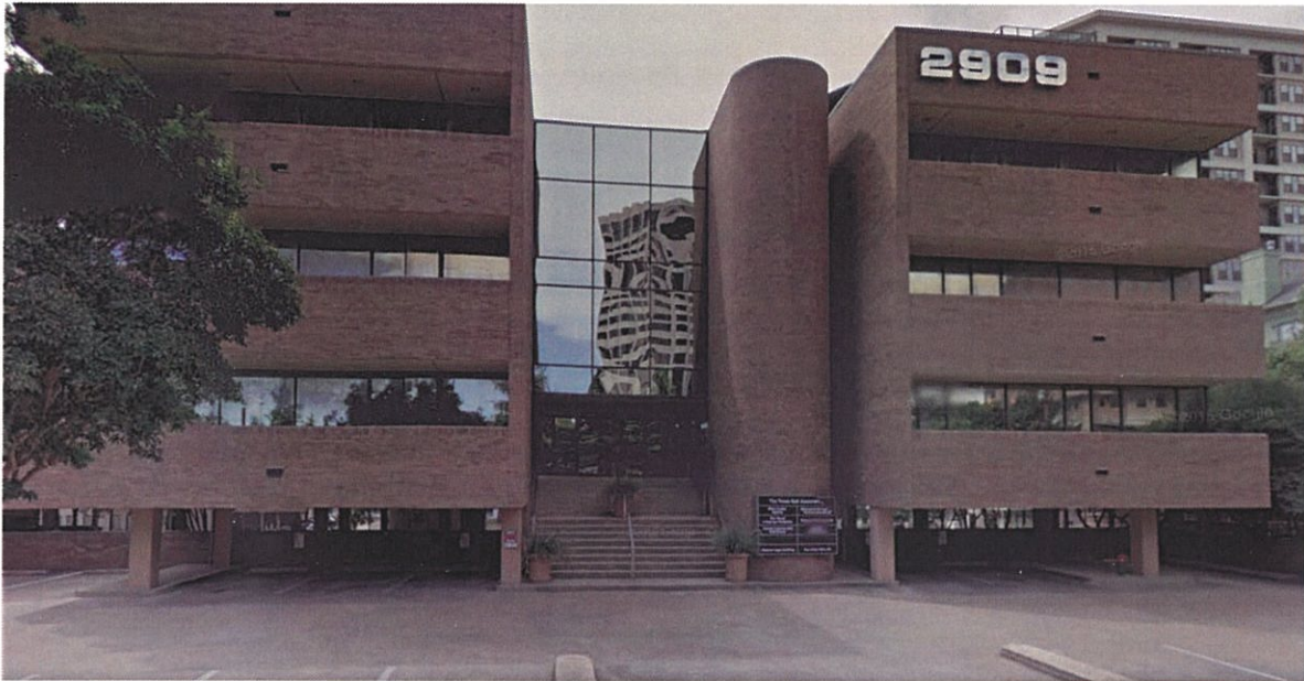
2909 Cole - First Floor Covered Parking
