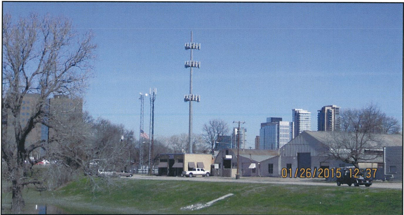
Extended 150' Monopole Tower
