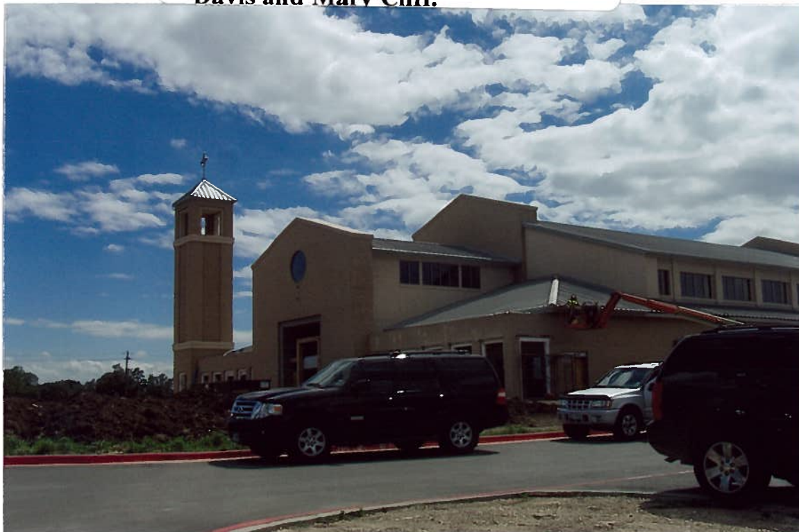
10. The new St. Cecilia Church under construction.
