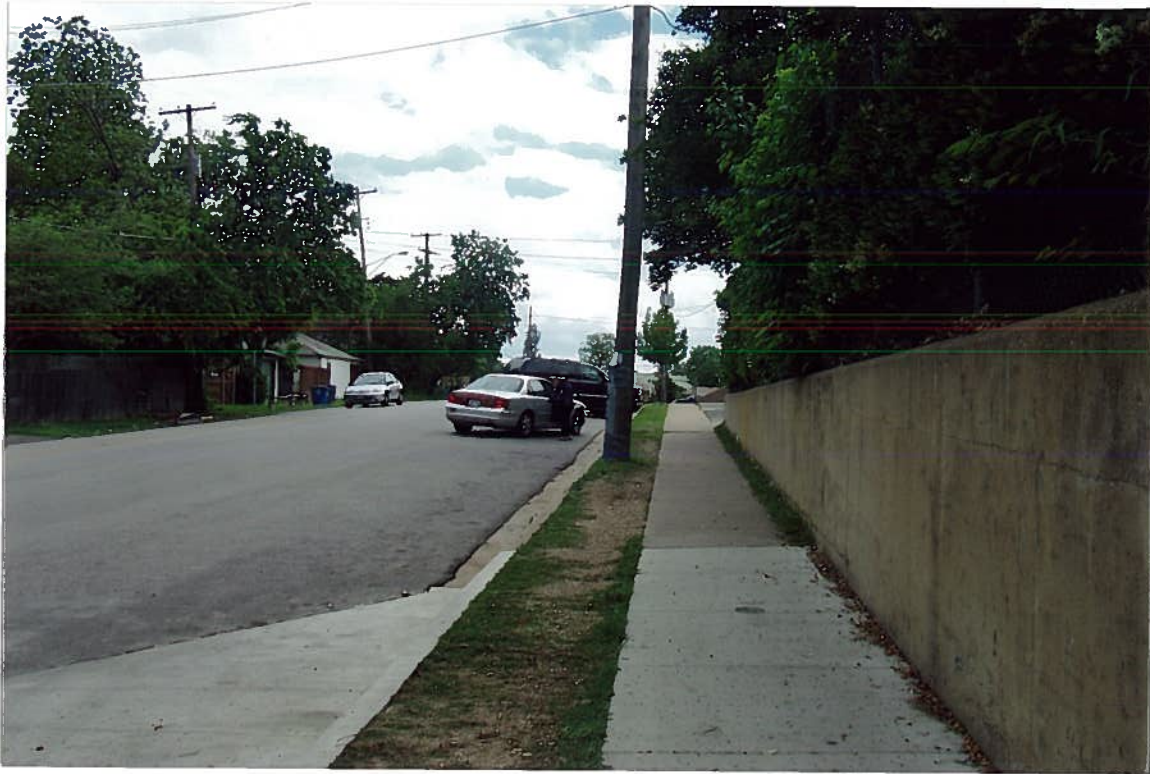
1. The sidewalk viewed south on Mary Cliff Drive. Note the concrete retaining wall.
