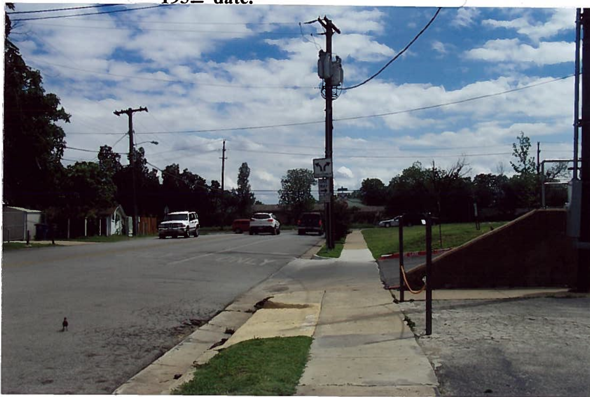
4. Continuation of the sidewalk to the intersection with West Davis Street.
