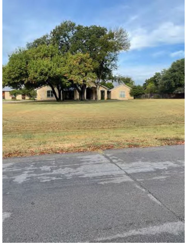
10625 Lennox, the house beside 10645 asking for the fence adjustment Open yard
