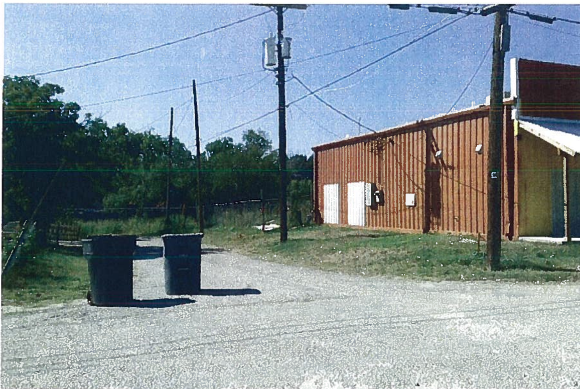
7. View of Pastor Street (dead-end street-site/building on right).
