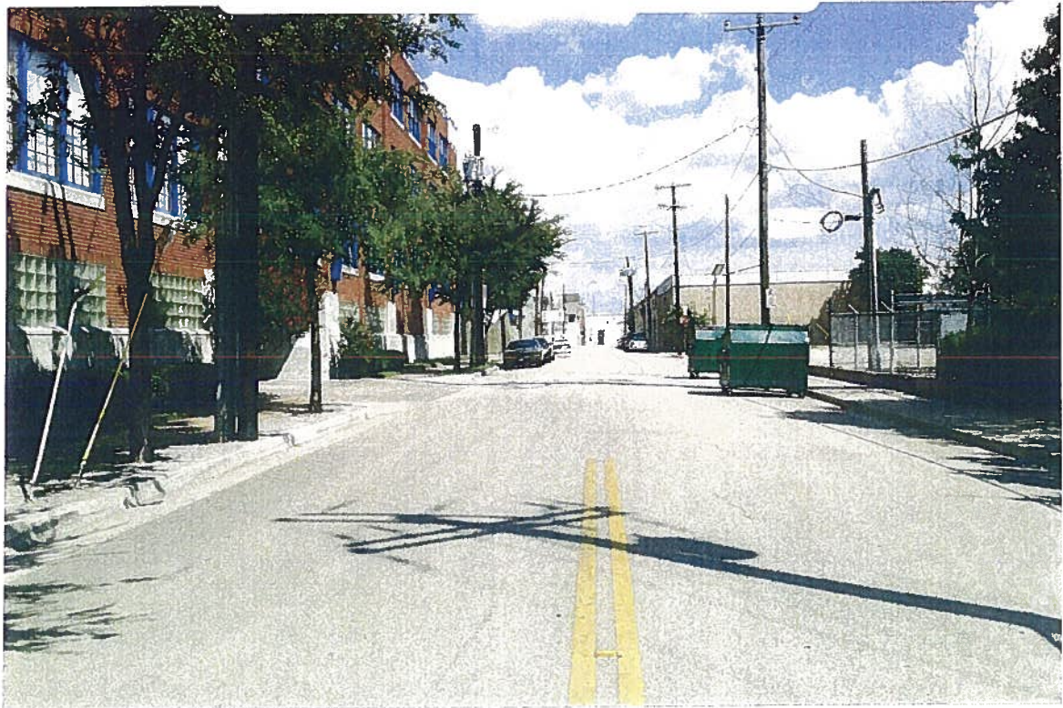
8. View south on Hawkins Street – site is on right (the dumpsters are not ours).
