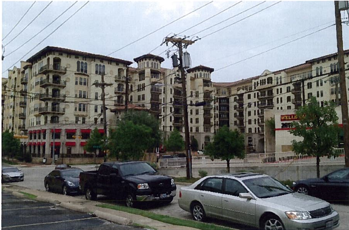
View of Gables Villa Rosa, across Carlisle Street from the site.
