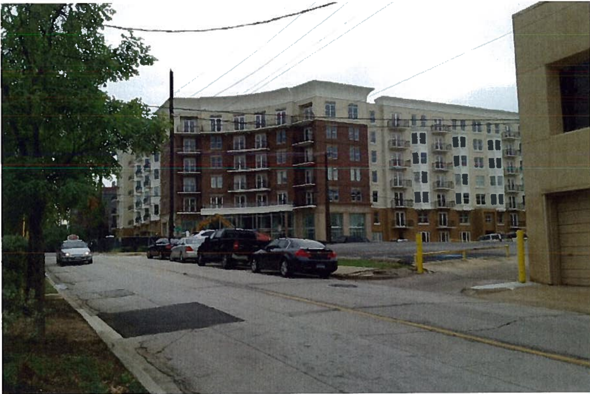
View of Gables project under construction (P.D. 193, P.D.S. 93)
